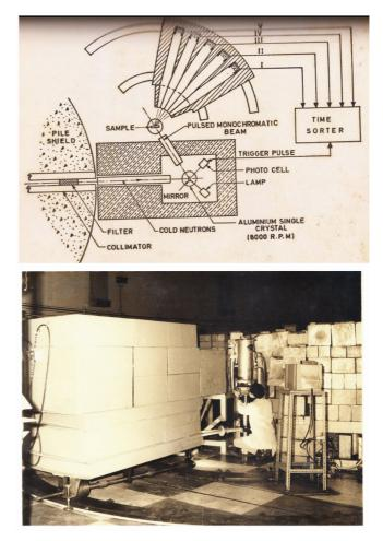
Figure 1. A schematic of rotating crystal spectrometer (top) and a photograph of the machine built by GV and Usha Deniz (bottom).
