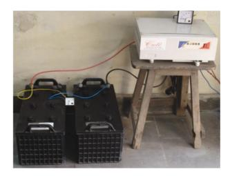
Figure 3. Solar inverter and battery backup of the SPV system.
