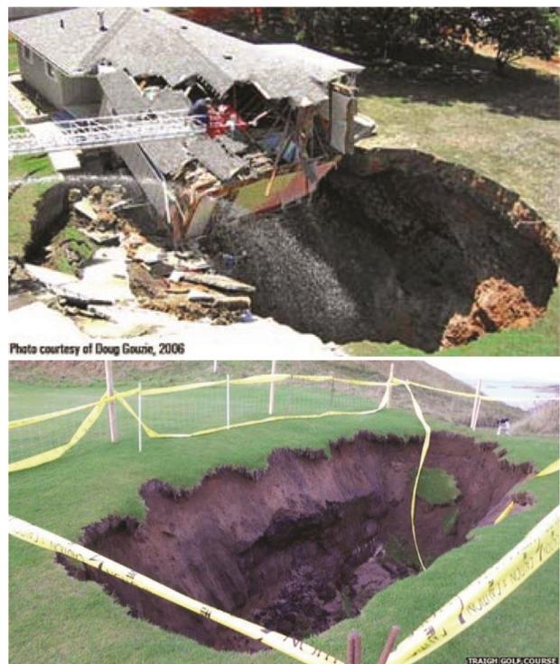
Figure 1. Impact of pot-hole subsidence on surface structure<sup>31,32</sup>.
