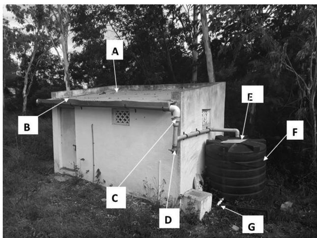
**Figure 1.** Installed RWH setup for an average-sized dwelling. A, Corrugated GI roof; B, Collection channel; C, SS mesh screen; D, First rainwater diverter valve; E, Cloth filter; F, Storage tank; G, Tap for drawing rainwater.
