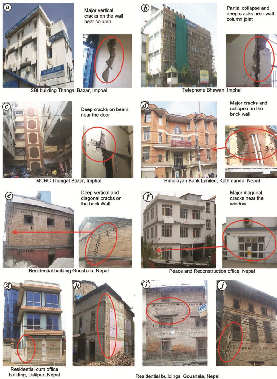
**Figure 2 a-j.** Damaged buildings during the Nepal earthquake 2015 and Imphal earthquake 2016.
