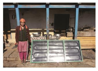
Figure 1. Mountain solar water-heating system in a rural household.
