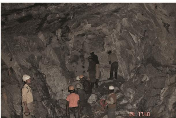
**Figure 8.** Loading of explosives in the sub-cycle I (pilot).
