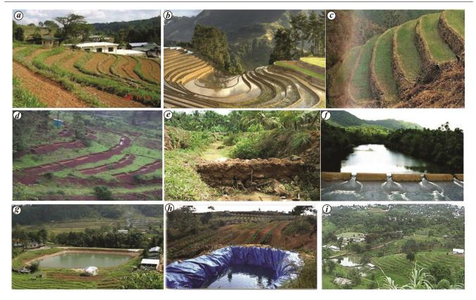
Figure 12. Soil and water conservation measures using structural/engineering methods such as (a) contouring, (b, c) bench terracing, (d) contour trench, (e) loose boulder check dam, (f) RCC check dam, (g) retention pond, (h) jalkund and (i) IFS. Photo courtesy: (a, e-i) ICAR Research Complex for NEH Region; (b) farmers of Meghalaya and (d) Low External Input Sustainable Agriculture, India.
