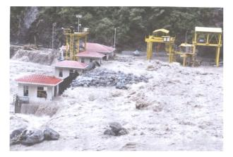
**Figure 9.** Flood filled the Alaknanda channel behind the Vishnuprayag dam with debris, inflicting crippling below to the project (courtesy: B. D. Patni).
