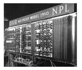
Figure 7. Pilot model of the automatic computing engine.
