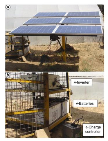
Figure 1. *a*, Solar modules of 600 W power pack system. *b*, View of inverter and batteries.
